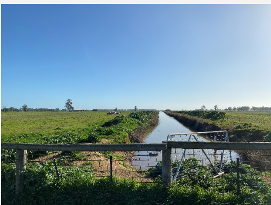
Figure 9: View north along irrigation channel – taken from existing bridge over channel
