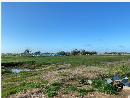
Figure 10: View southeast – taken from existing bridge over channel
