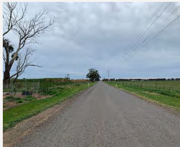
Figure 11 Broockmanns Road looking west.
