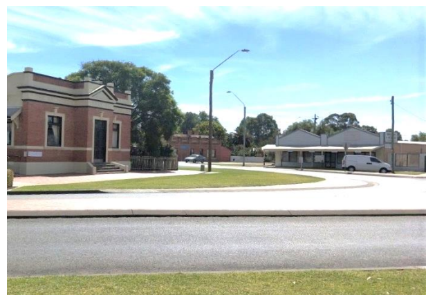
Photo 12: West view of Murray St facade
