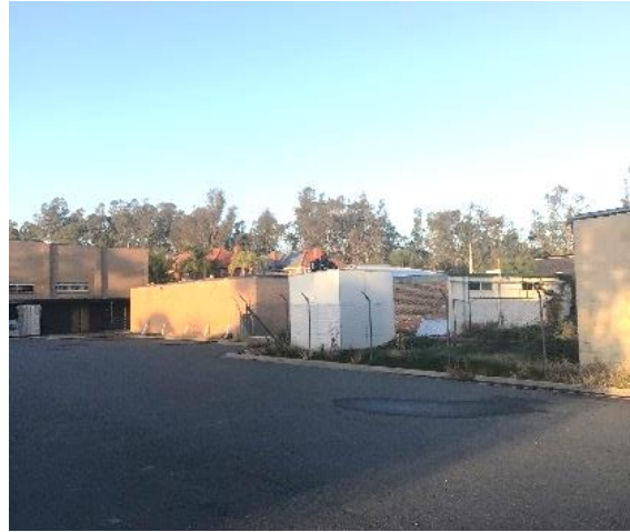
Photo 20: East view of hardware & motel building facades
