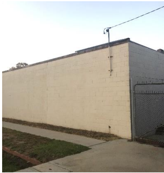
Photo 16: View of later rear building north facade
