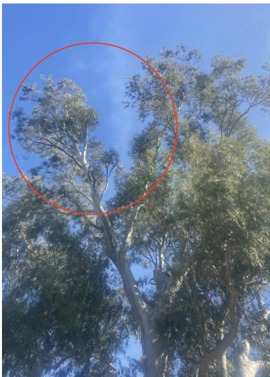
Figure 10: Upper canopy tree #1 exhibits previous failures
