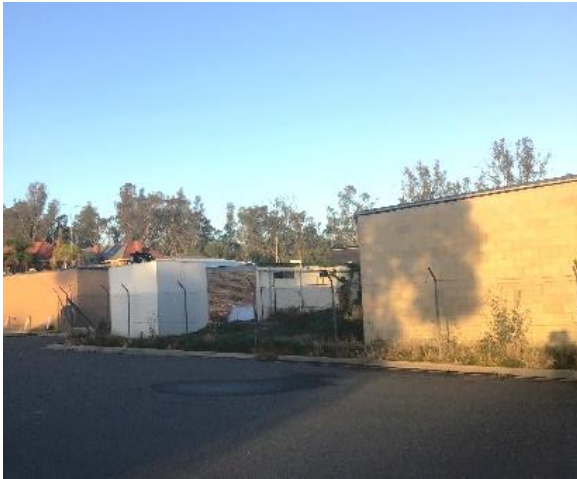
Photo 19: East view of later rear building façade
