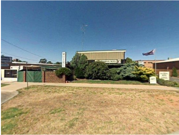
Photo 1: West view of Murray street 2 storey façade
