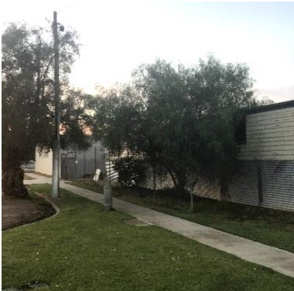
Photo 15: View of part north façade (rear)
