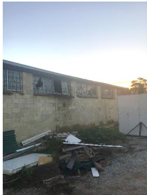
Photo 22: South view of later rear building façade
