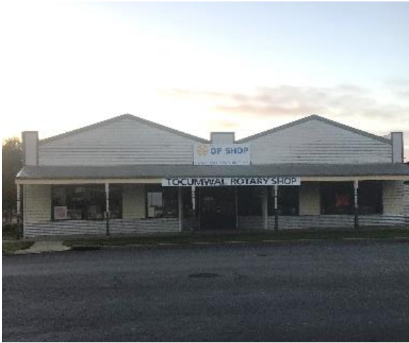
Photo 13: View of Murray St west façade & verandah
