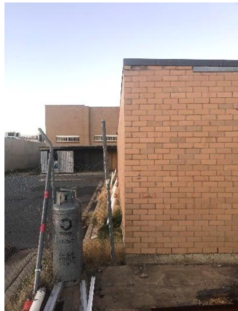
Photo 24: View of yard and north wall of motel facade
