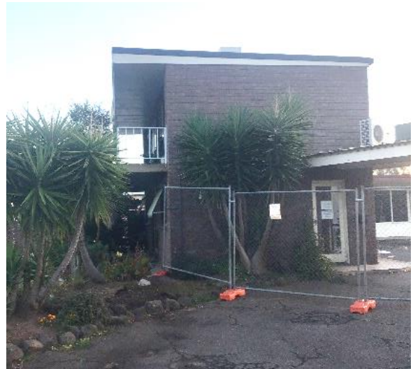
Photo 4: View of reception & 2 storey façade
