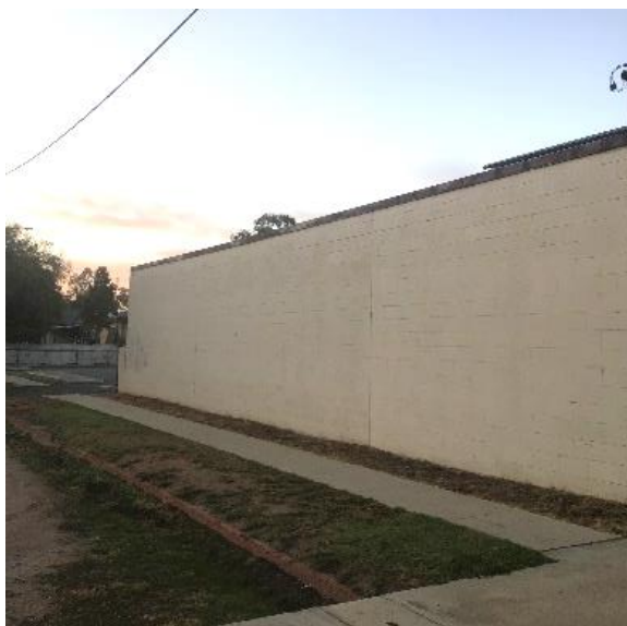
Photo 17: View of later rear building north facade
