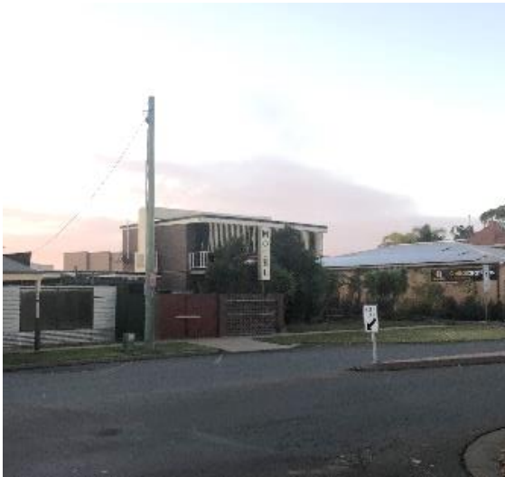
Photo 3: NW view of Murray street 2 storey façade
