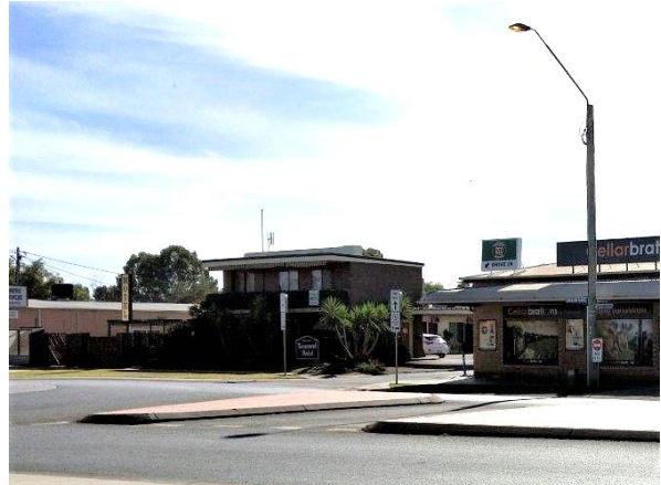
Photo 2: SW view of Murray street 2 storey façade
