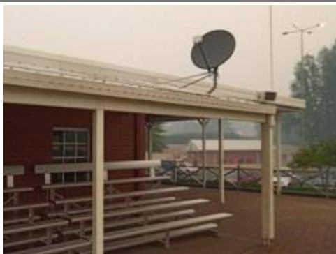
Figure 1: Sky Muster antennae installed on roof
