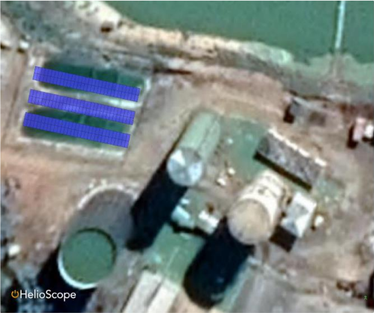
Finley Water Treatment Plant - 83.7kW- Solar PV + BESS - Ground - STC
