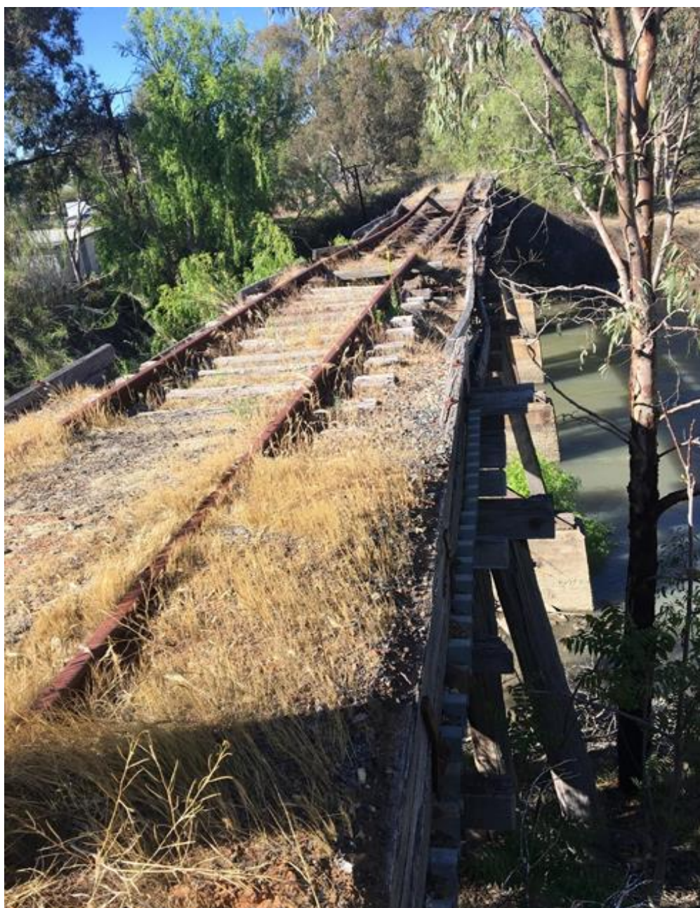
Figure 4 – Typical Timber Ballast Deck Structure
