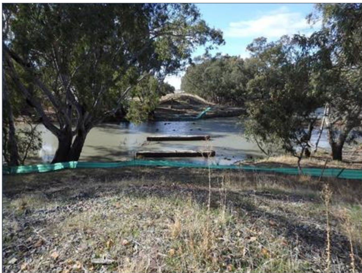
Figure 3 - Removed Underbridge over Billabong Creek, Jerilderie
