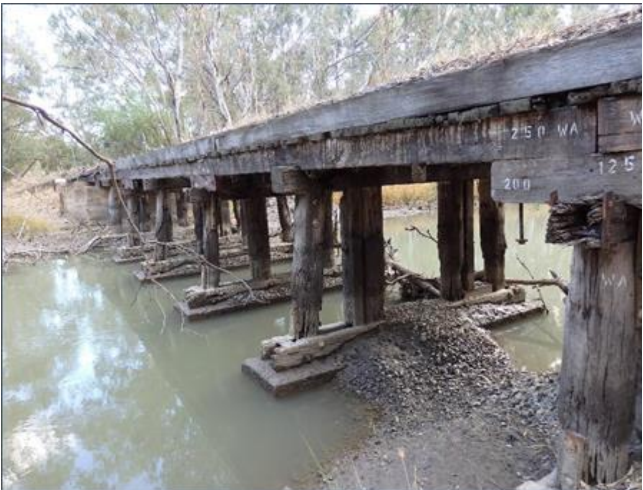
Figure 6 - Underbridge over Morundah Creek, Morundah
