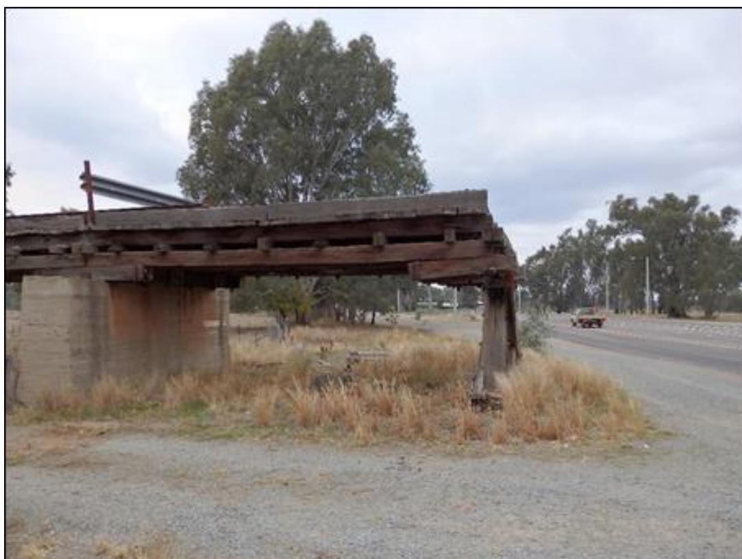
Figure 5 - Viaduct No. 2 (spans removed over the Sturt Highway)
