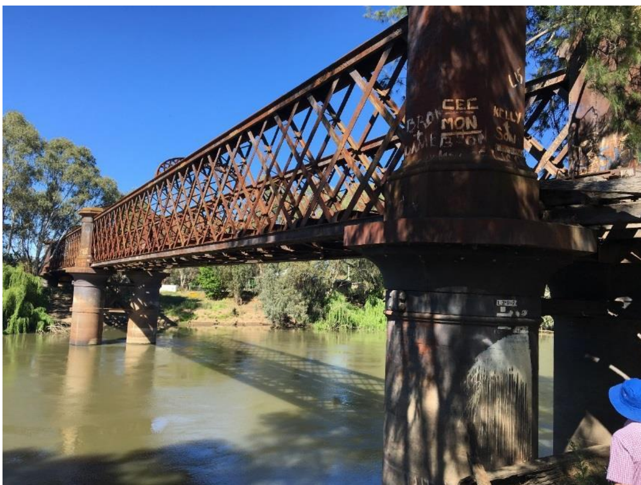
Figure 1 – Narrandera Truss Bridge across the Murrumbidgee
