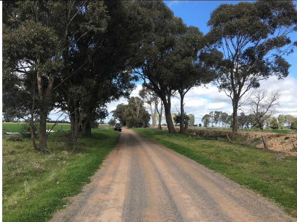
Disturbed edges of the road showing the heavy loads of pasture grasses.
