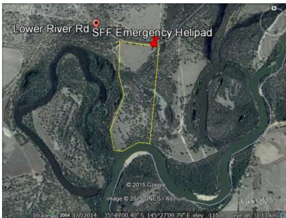
General satellite view of the proposed venue site.
