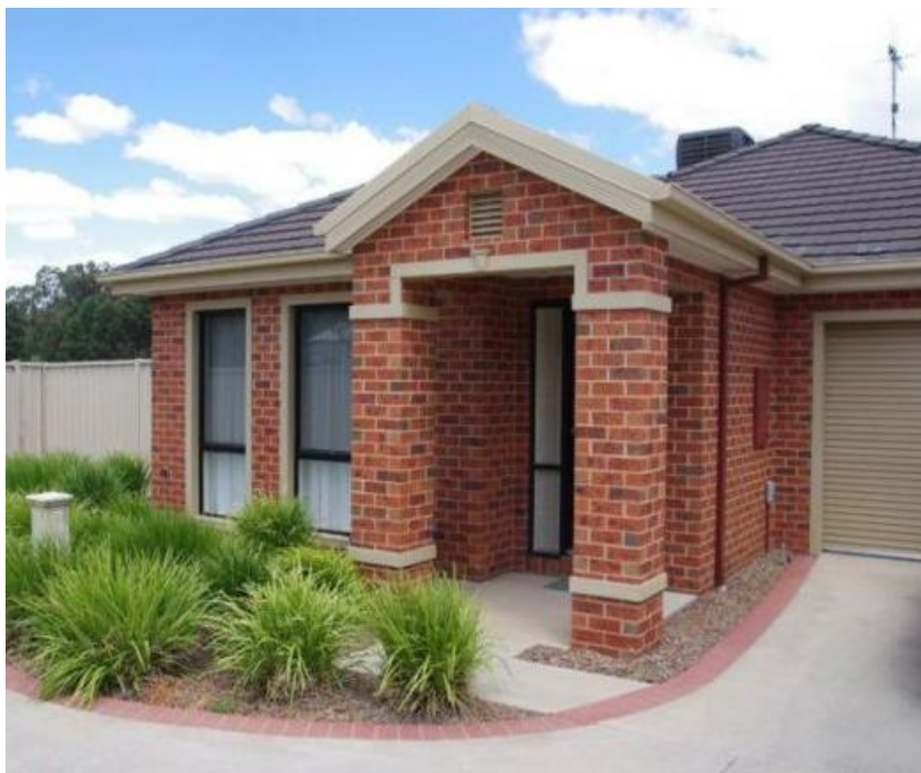
Photograph 1: New housing at Tocumwal (image courtesy of Domain.com.au)
