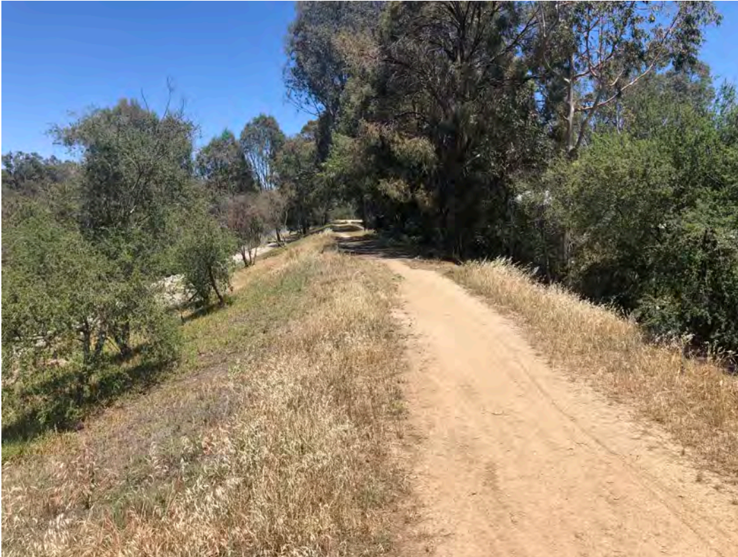
Photo 3: East end of levee strengthening works, west orientation. Works are to consist of a 3.5m deep trench in the top of the levee filled fill concrete and back-filled. Photo: D.Wall
