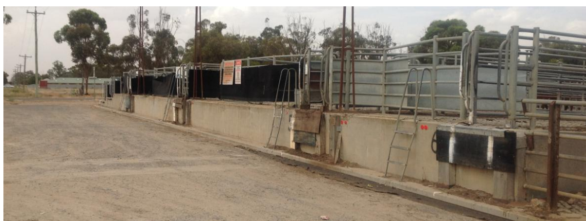
Pic Above- Current ramp loading docks
