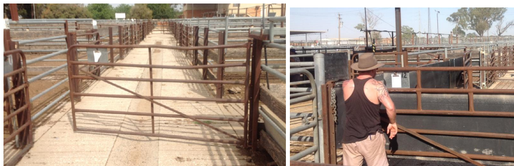
Pic Above- Gate not long enough to cross lane
