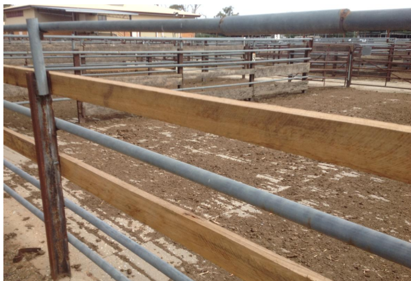
Pic Above- Typical Fence
