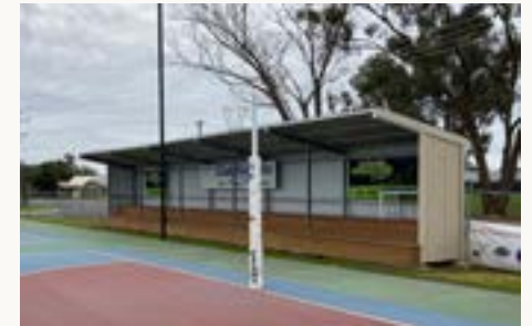
Covered seating along netball courts.
