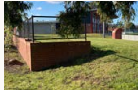
Retaining wall at rear of spectator grass mound.
