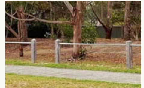
Bollard and rail vehicle restriction barrier.
