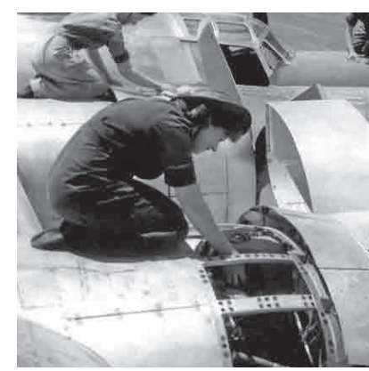
Fitting to suit WWII air base construction techniques
