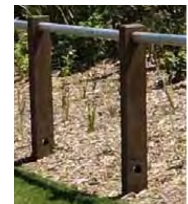
Bollard and pipe fence with timber bollard Finish Hard wood Galv pipe
