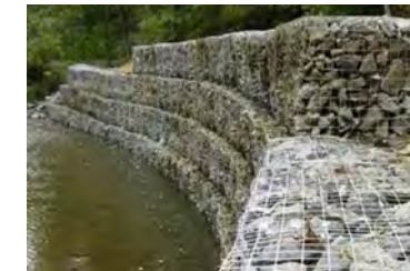
Gabion basket retaining wall
