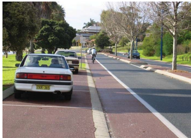
Town of East Fremantle, Western Australia
