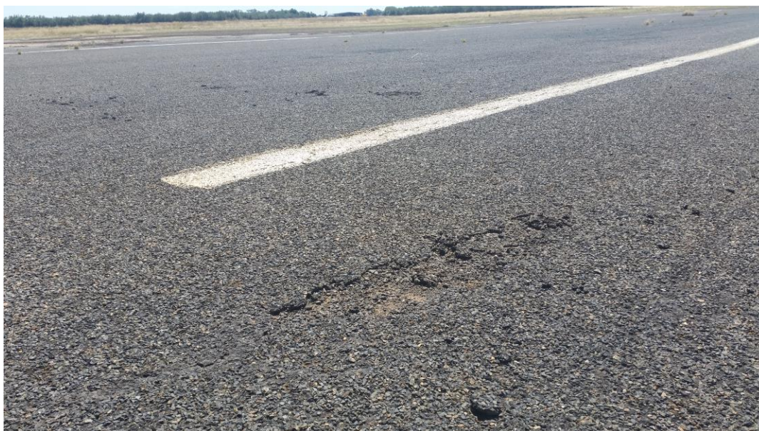
Typical Cracking over failing Pavement – Runway 18-36
