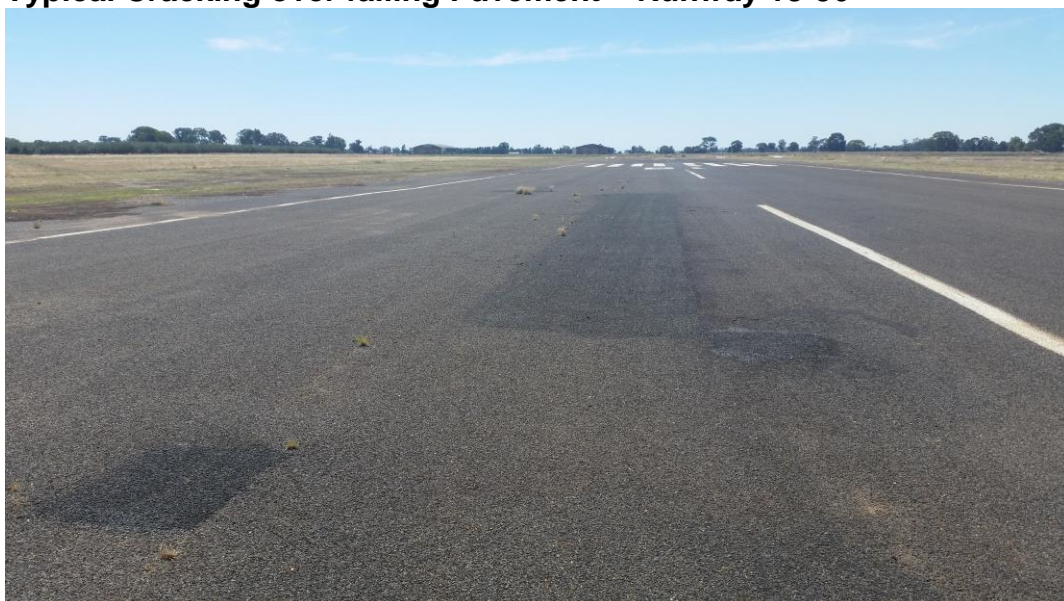
Typical Cracking over failing Pavement – Runway 18-36
