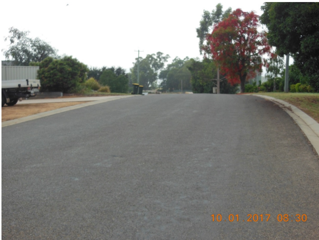
Figure 15- Photo taken in Dip with camera at breast height (note you cannot see wheelie bins)
