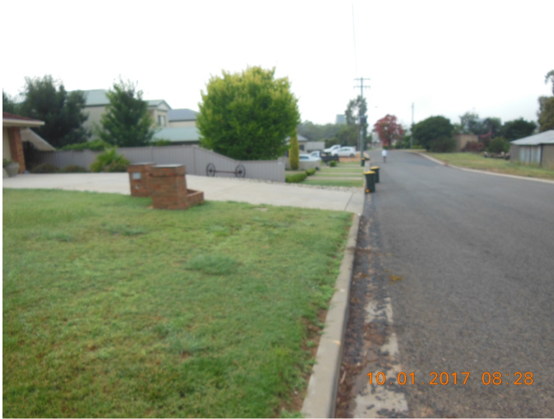
Figure 6- Steep driveways to match footpath
