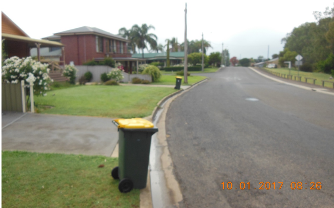
Figure 23- Obstacles north side
