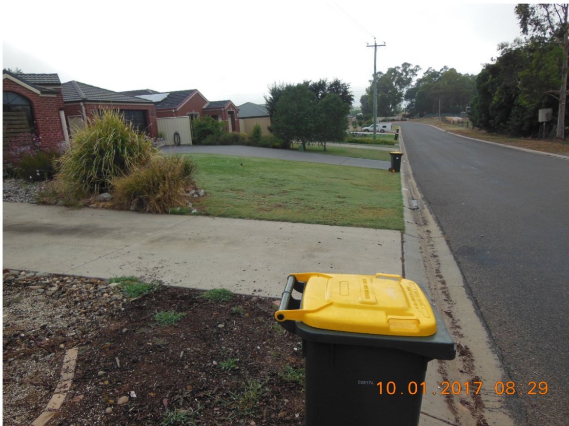
Figure 9- Steep driveways to match footpath
