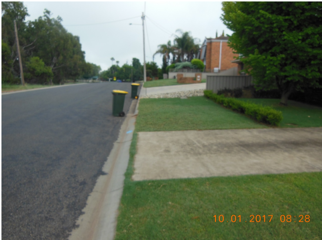
Figure 7- Steep driveways to match footpath
