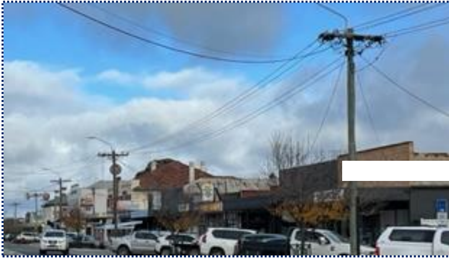
Figure 1: Existing overhead powerlines with crossings
