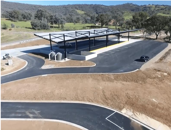
Figure 5: Drop off facility for heavy and Construction Waste
