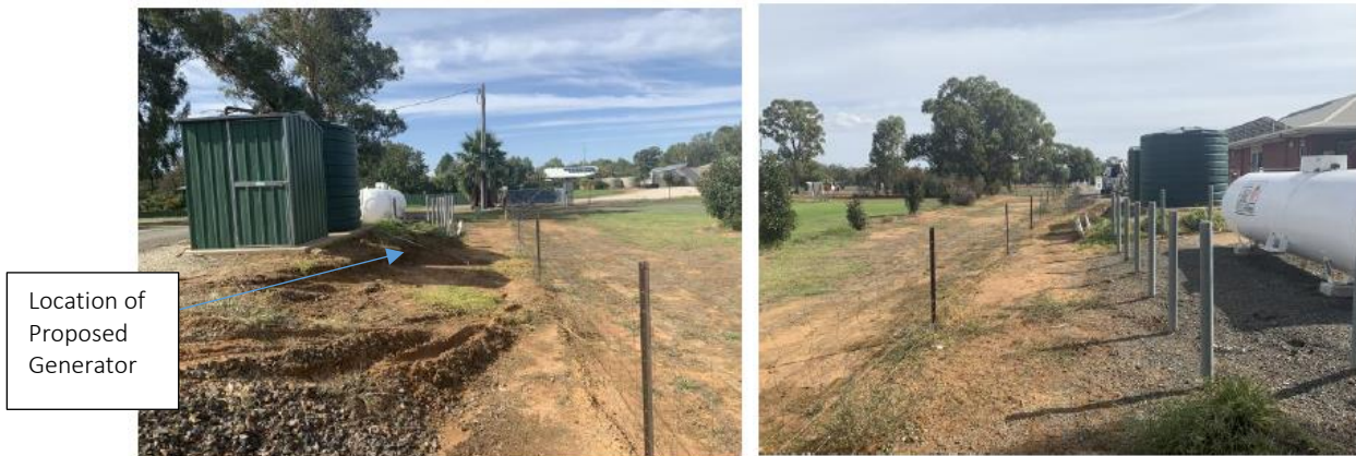
Figure 4 and 5 – existing site conditions and location for proposed Generator
