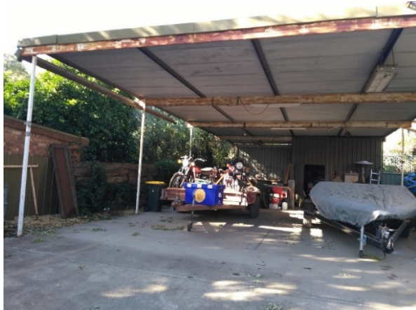
Figure 7 – street view of the location of the proposed carport
