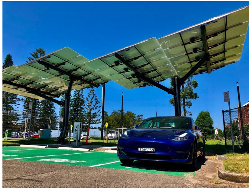
Example of shade structure with solar panels
