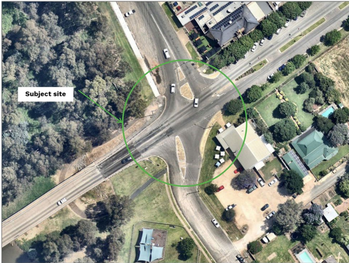
Figure 2: Aerial image of the site (reproduced from Nearmap)
